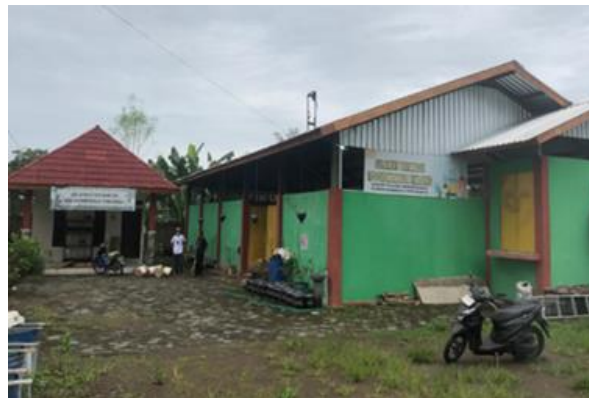
Gambar 2. Gedung TPS3R Nirmala Tanjung
